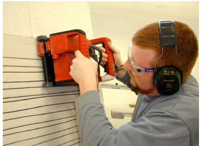
Wall chaser used for cutting grooves in sand-lime brick
